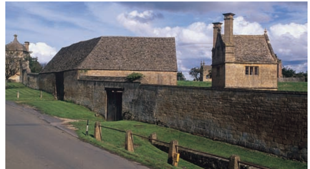
Court Barn in Church Street, Chipping Campden
